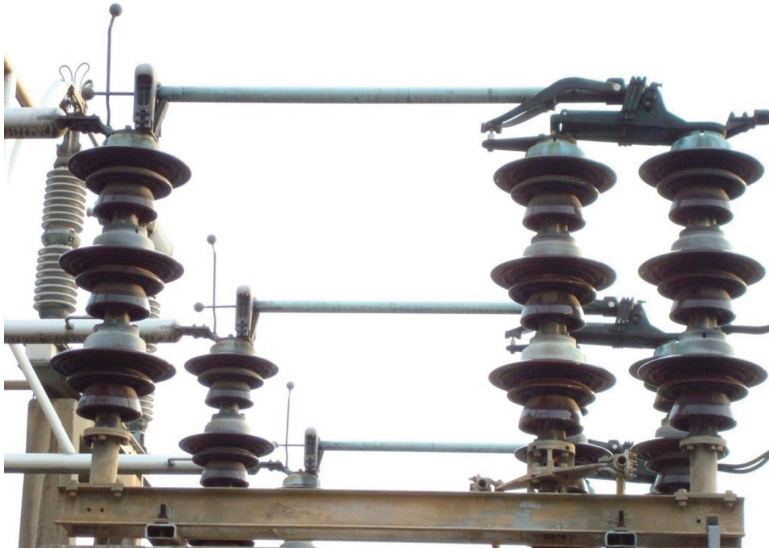
Figure 2.23 Disconnect switch.
