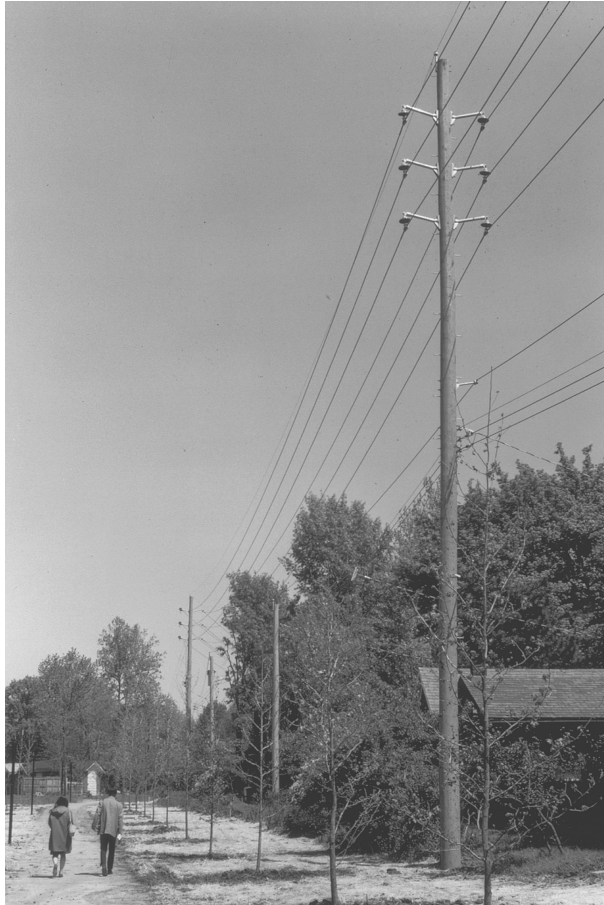
Figure 2.32 A typical 34.5 kV line with a double circuit and wood poles. It has a newer style construction. (Union Electric Company.)
