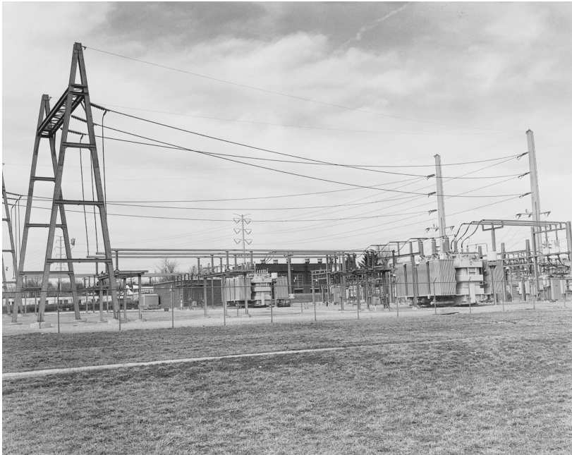
Figure 2.37 A bulk power substation operating at 138/34.5 kV voltage level. (Union Electric Company.)
