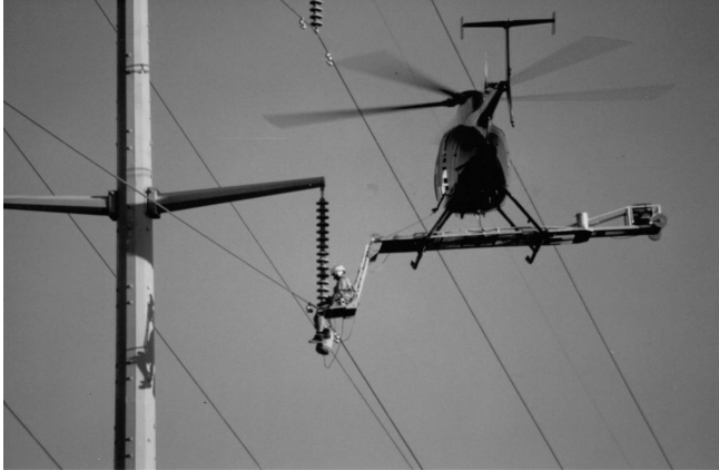
Figure 2.15 A lineman working from a helicopter platform.
