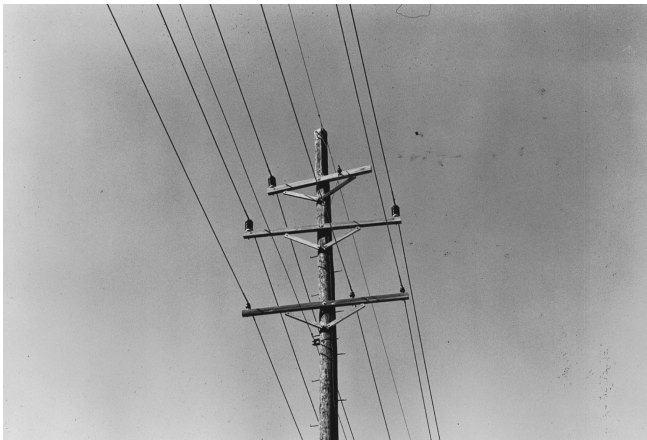
Figure 2.33 A 34.5 kV line with a single circuit and wood poles. It also has a 12.47 kV underbuilt line and 34.5 kV switch. It has an old style construction. (Union Electric Company.)
