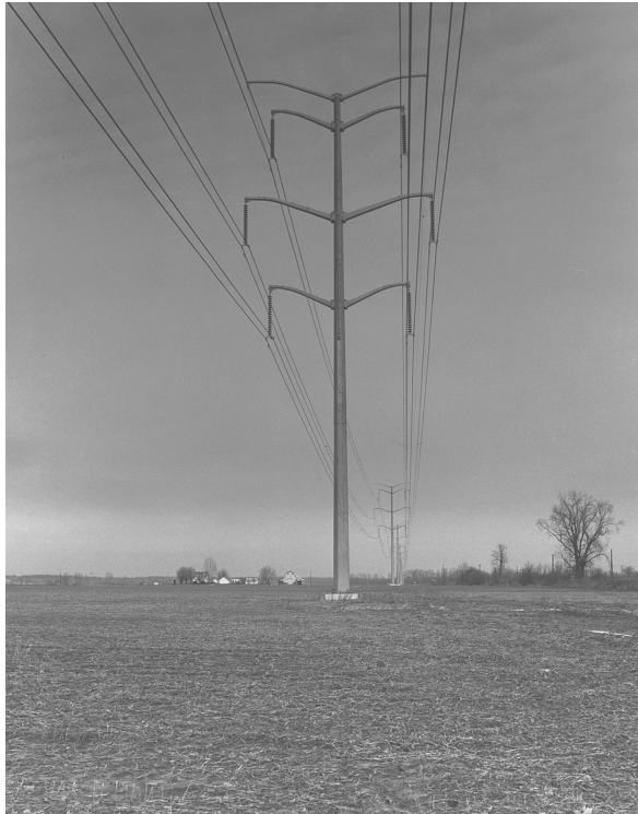
Figure 2.8 A typical 345 kV transmission line with bundled conductors and double circuit on steel towers. (Union Electric Company.)
