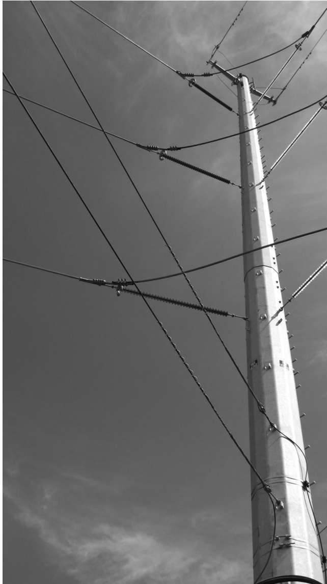
Figure 2.26 A galvanized dead-end corner pole of a 230 kV transmission line. (Courtesy of West Power Inc.)
